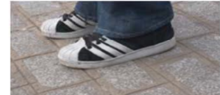
Flush, fine picked granite setts suitable for walking
