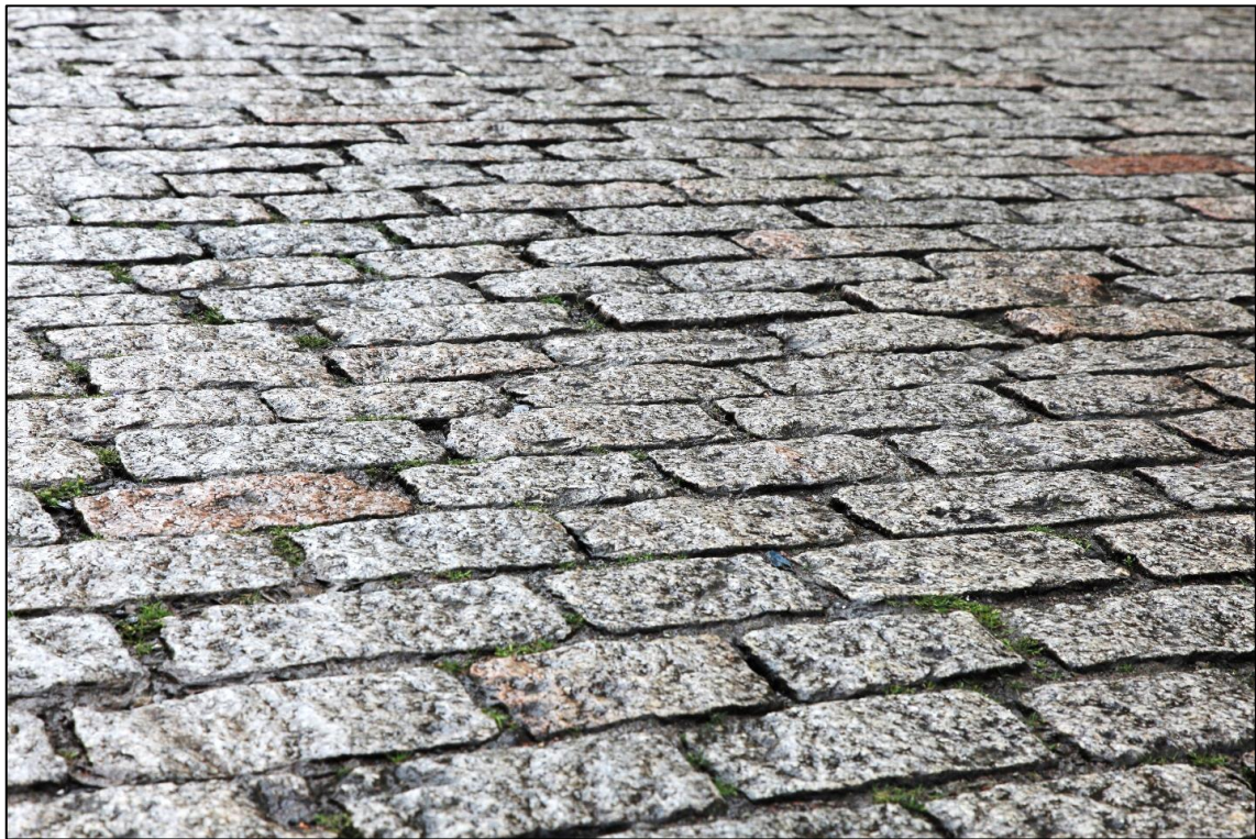
Figure 2 Typical character of a traditional setted street in Edinburgh
